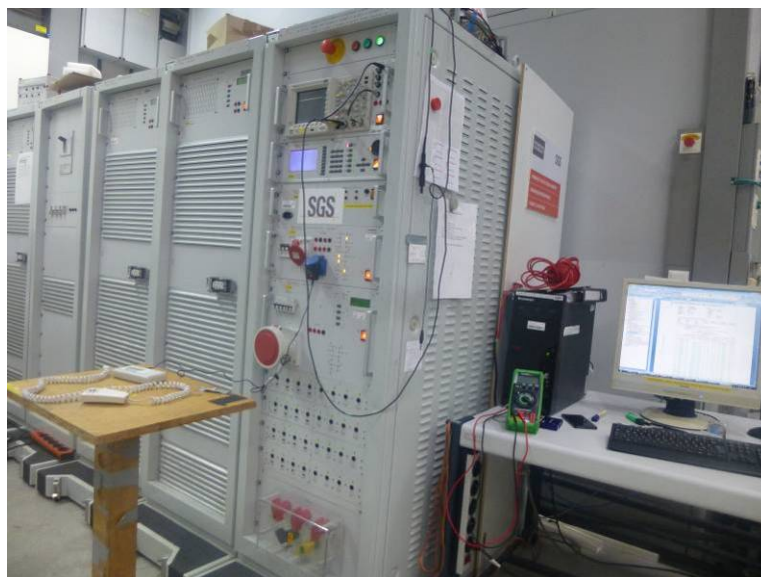
Figure 6-12: test setup for harmonic current emissions
